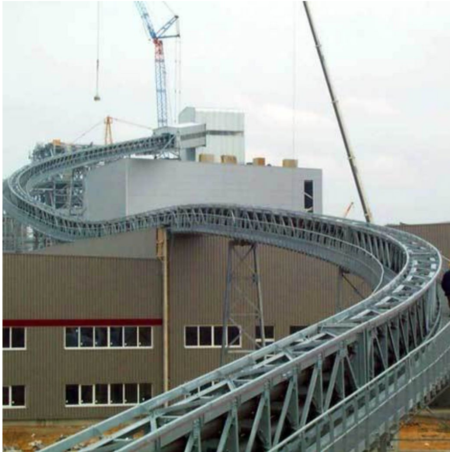
Figure 3. Example of a pipe conveyor, providing enclosed ore transport and flexible routing
