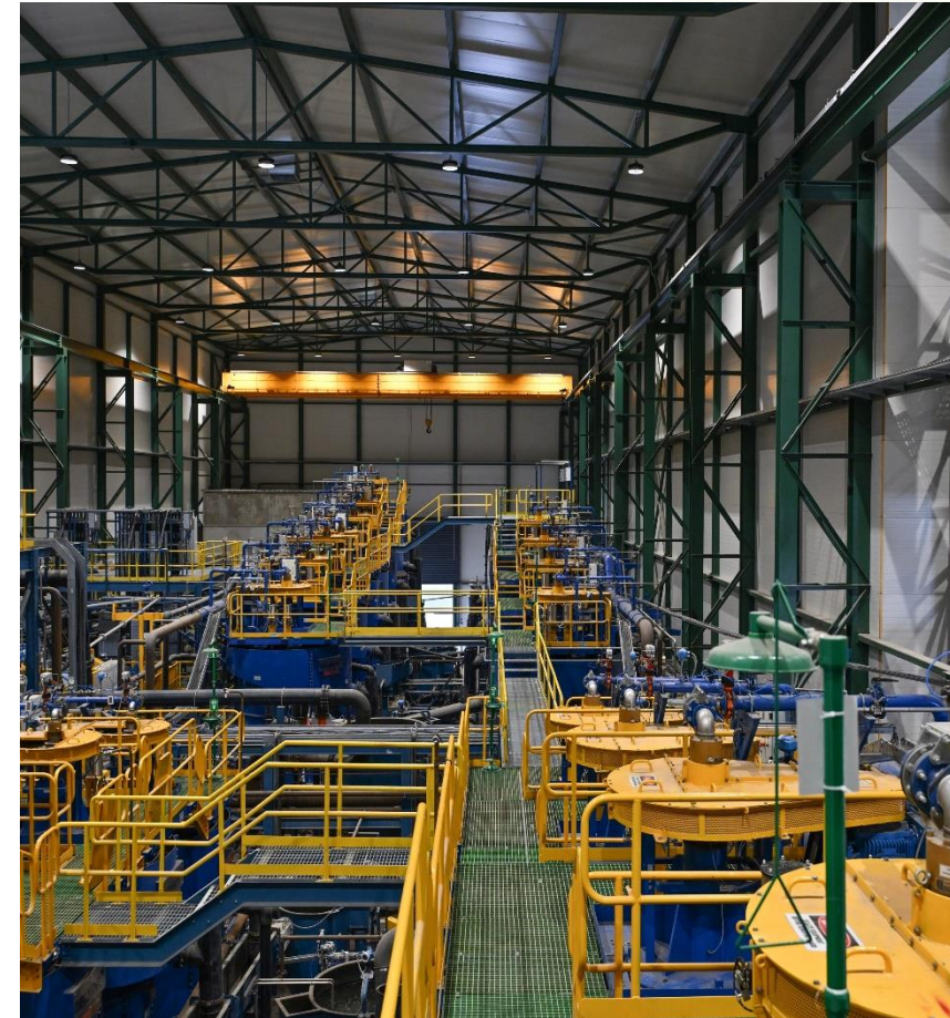
Vares Processing Plant, Aug 2024
