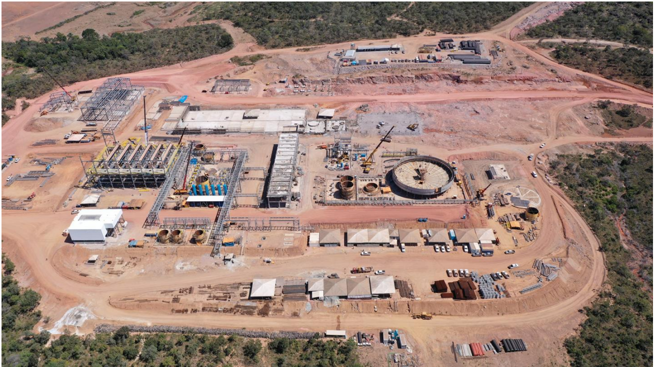
Figure 6: Serra Verde plant construction (taken in May 2022).
