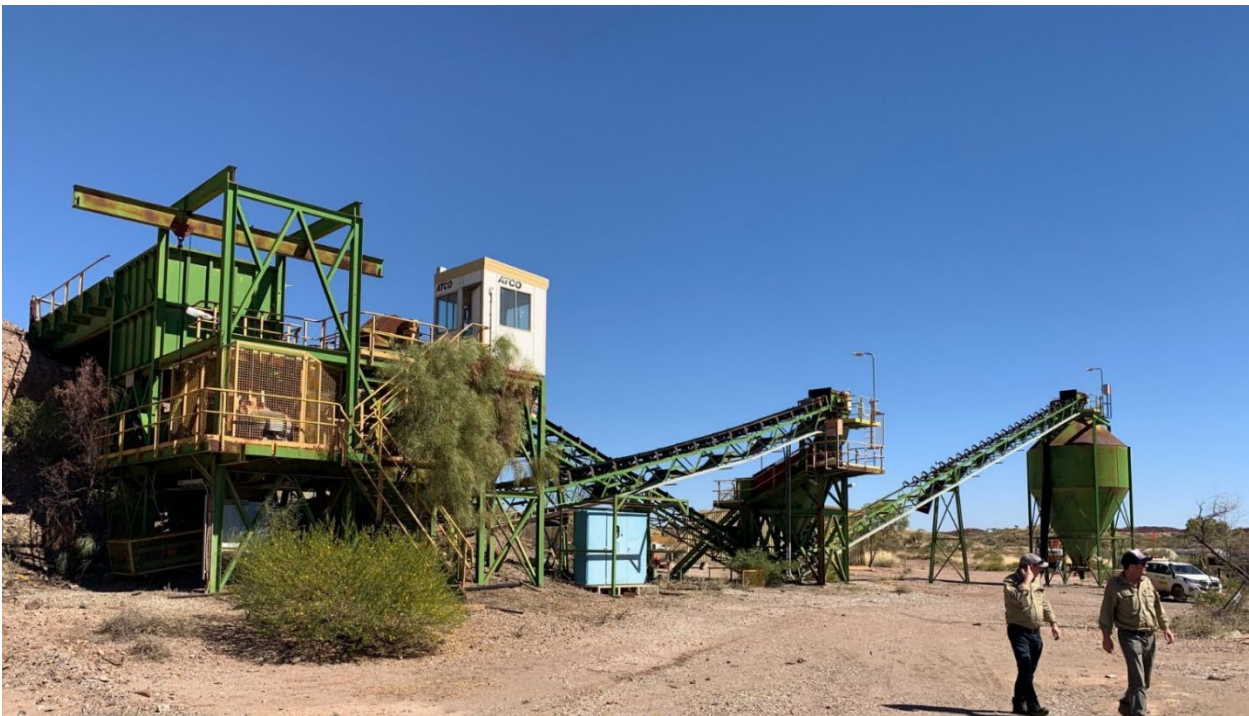
Figure 8: Existing Crushing Plant at Blue Spec
