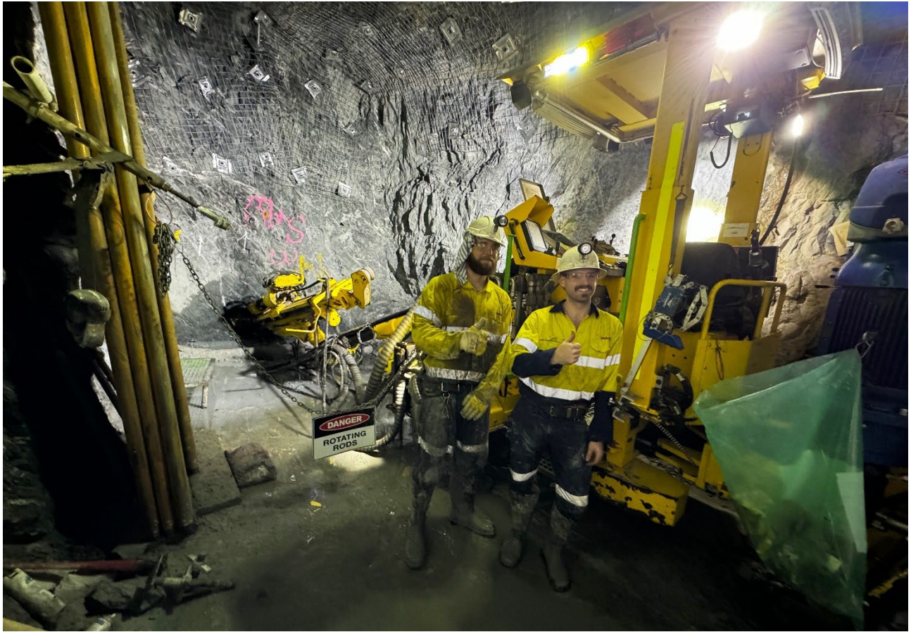
Figure 2: Diamond drill rig mobilised and drilling commenced
