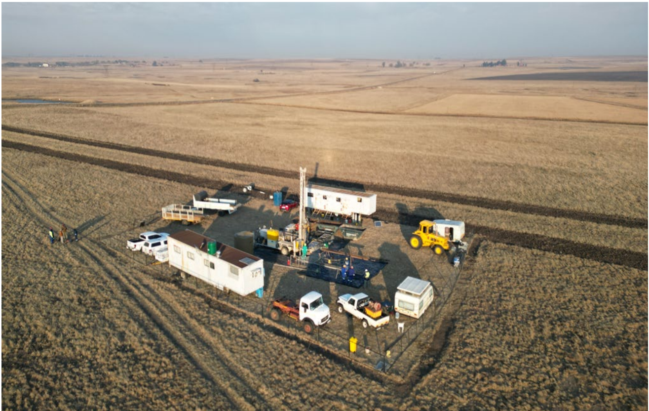
Figure 1: Drilling operations at core well ER272-06C
