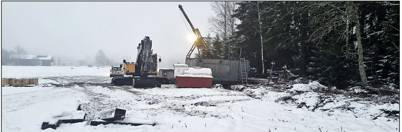
Figure 3: Drilling during the winter months at Granmuren.
