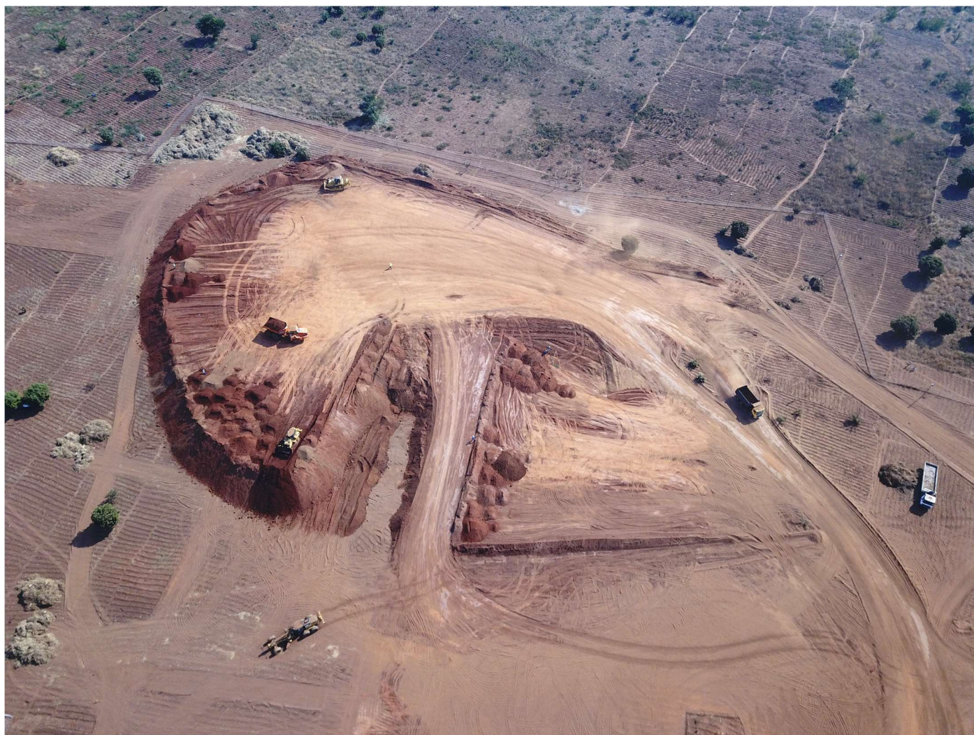
Figure 2: Dry mining stockpile area under construction
