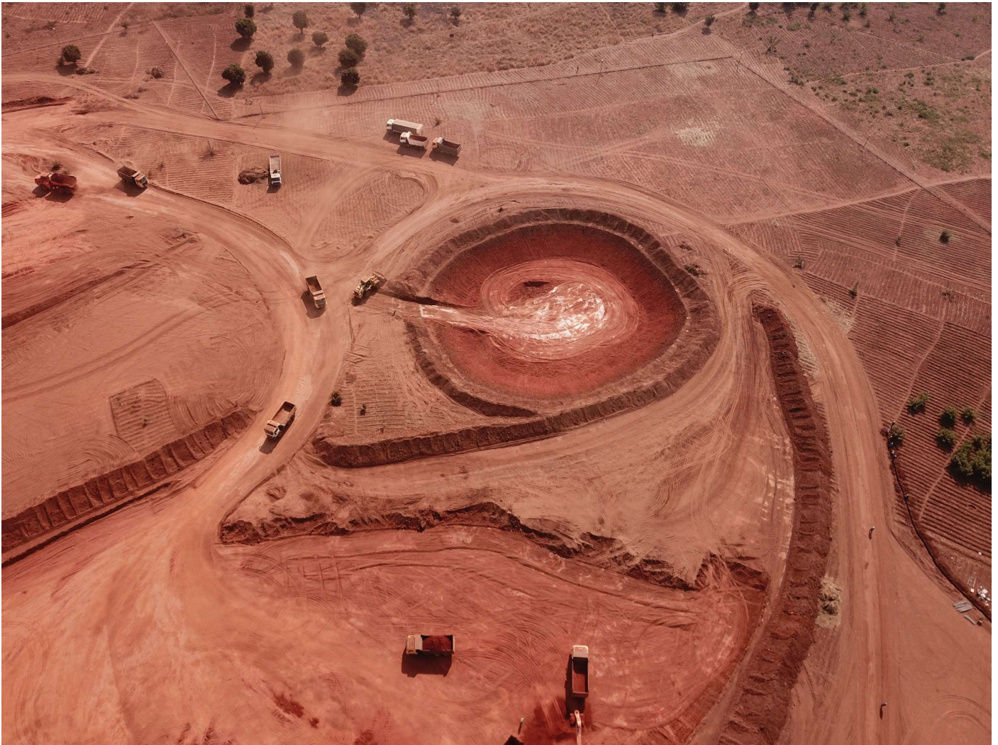
Figure 3: Pilot Phase fleet and equipment excavating the water storage pond
