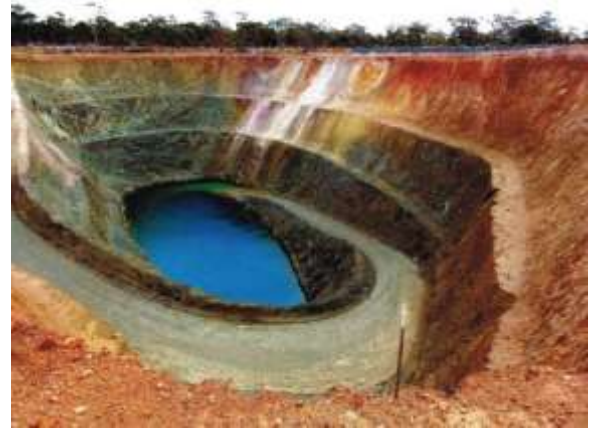
Figure c - HHH open cut
