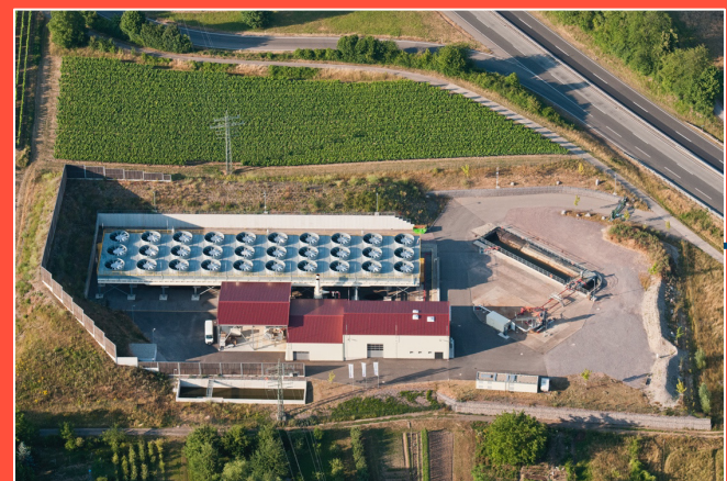
Geothermal Plant Insheim (A1)
